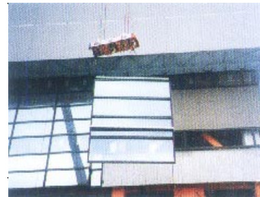
Fig.5 Unitized glass curtain wall
