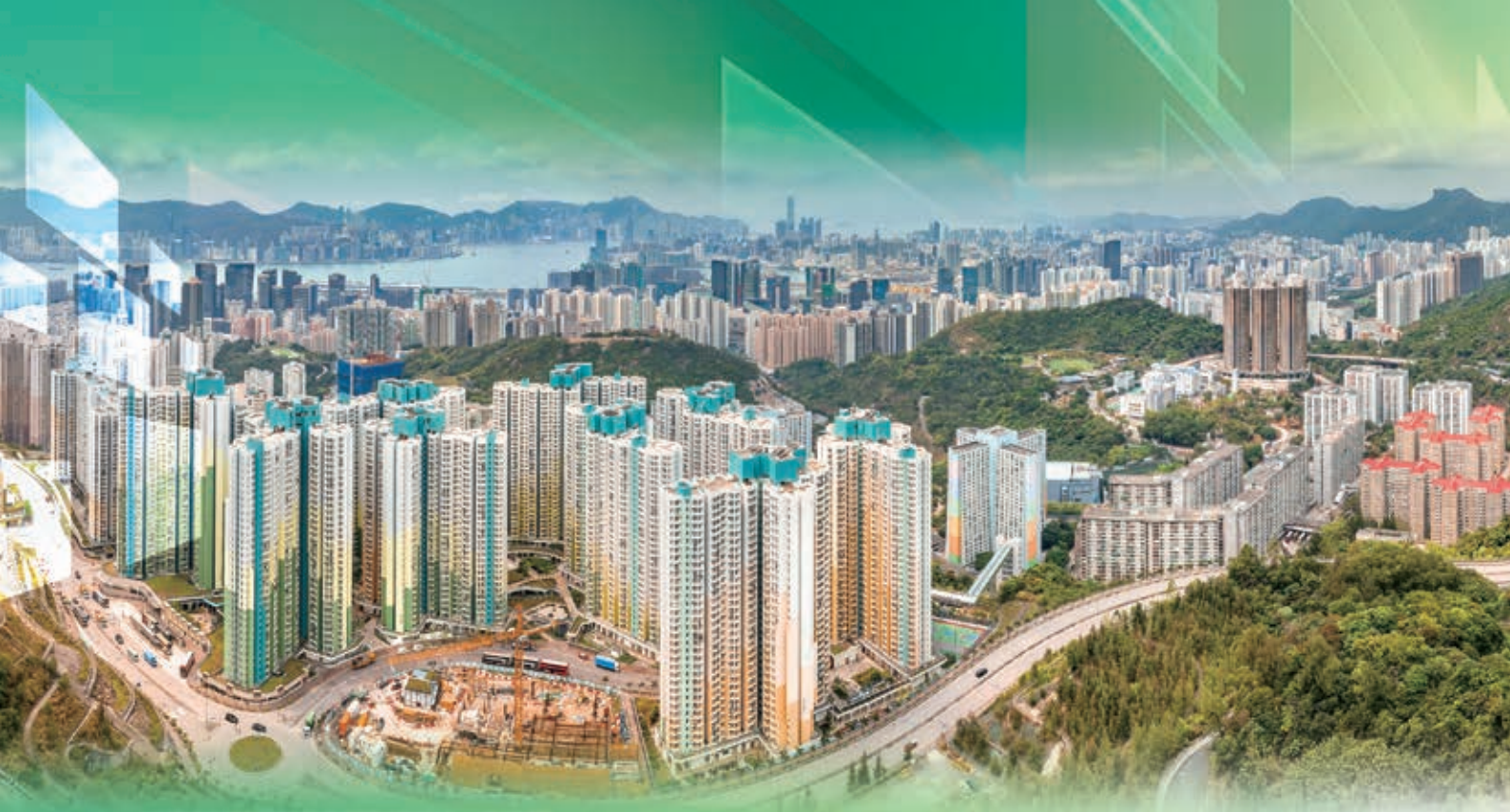
观塘安达臣道公营房屋发展项目 — 安泰邨 A public housing development at Anderson Road, Kwun Tong – On Tai Estate
