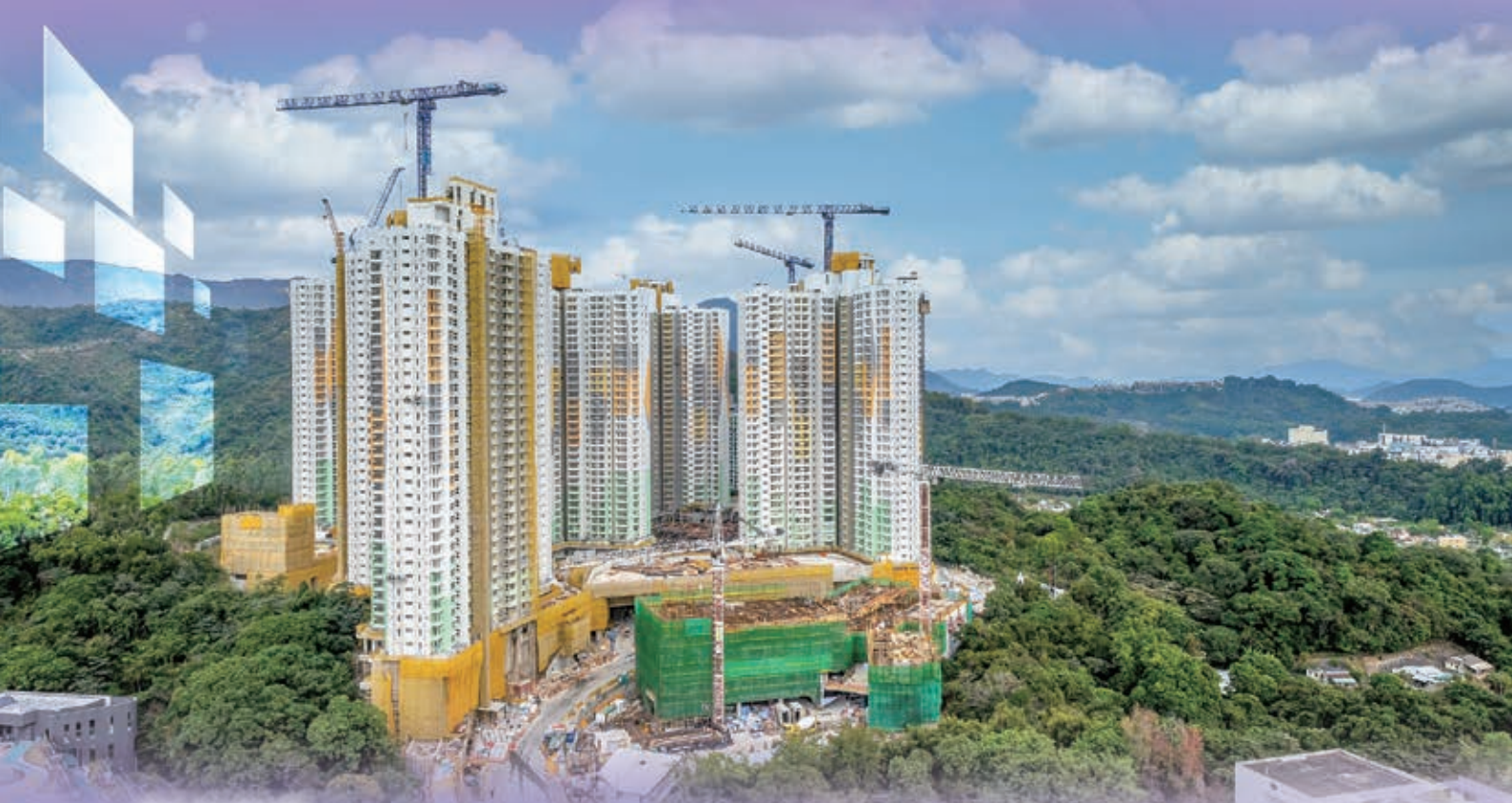
兴建中的富蝶邨 Fu Tip Estate under construction
