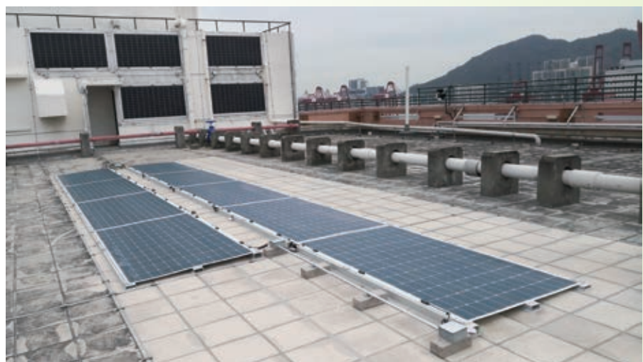
荔景邨的柔性太阳能光伏系统 A flexible PV system at Lai King Estate
