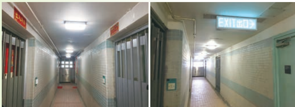
发光二极管凸面照明器 (左图)和出口指示牌 LED bulkheads (left photo) and an LED exit sign
