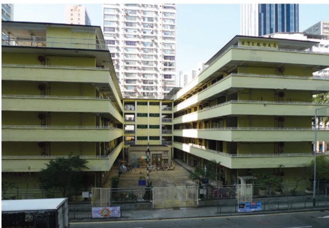
Chai Wan Flatted Factory - Before Conversion
