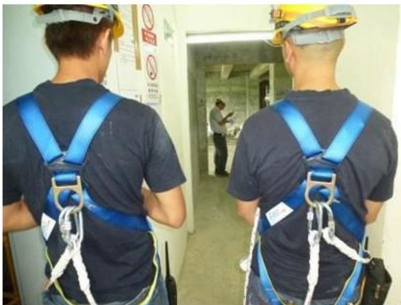
Workers Wearing PPE on Site 正确使用个人防护装备
