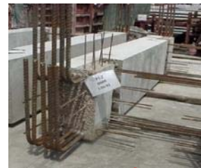
Precast Tie Beams
