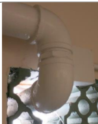
Disturbed grille panel
