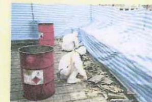
▲ Workers are carefully removing asbestos containing roof tiles
