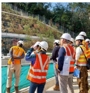
Joint inspection of the slope under construction conducted by HA and CEDD professionals.
