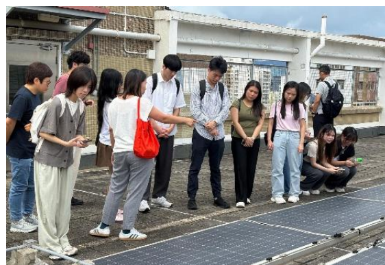
A visit to the solar photovoltaic system in Lok Wah North Estate arranged by EMD.
