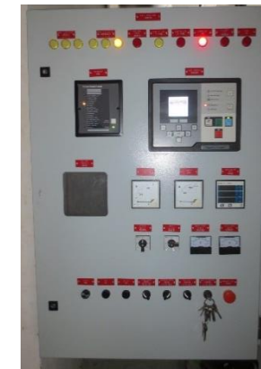
Emergency Generator, Control Cubicle and Switchgear Assembly
