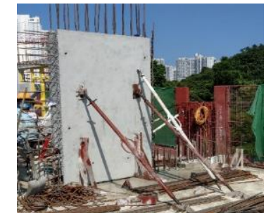
Precast Structural Wall (with concealed conduit)
