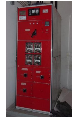
Emergency Generator, Control Cubicle and Switchgear Assembly
