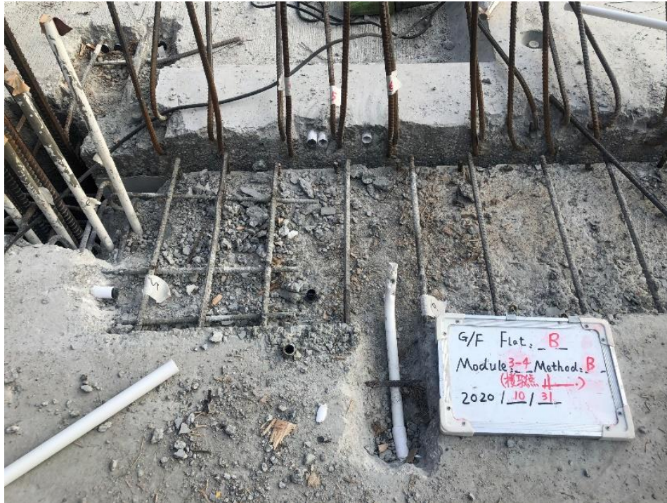
MiC Modules Assembly before conduit connection
