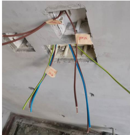
Cables with identification labelling
