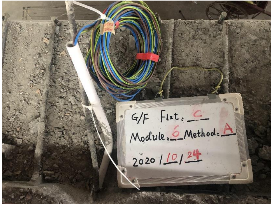
Cable reserved above the slab at temporary recessed area
