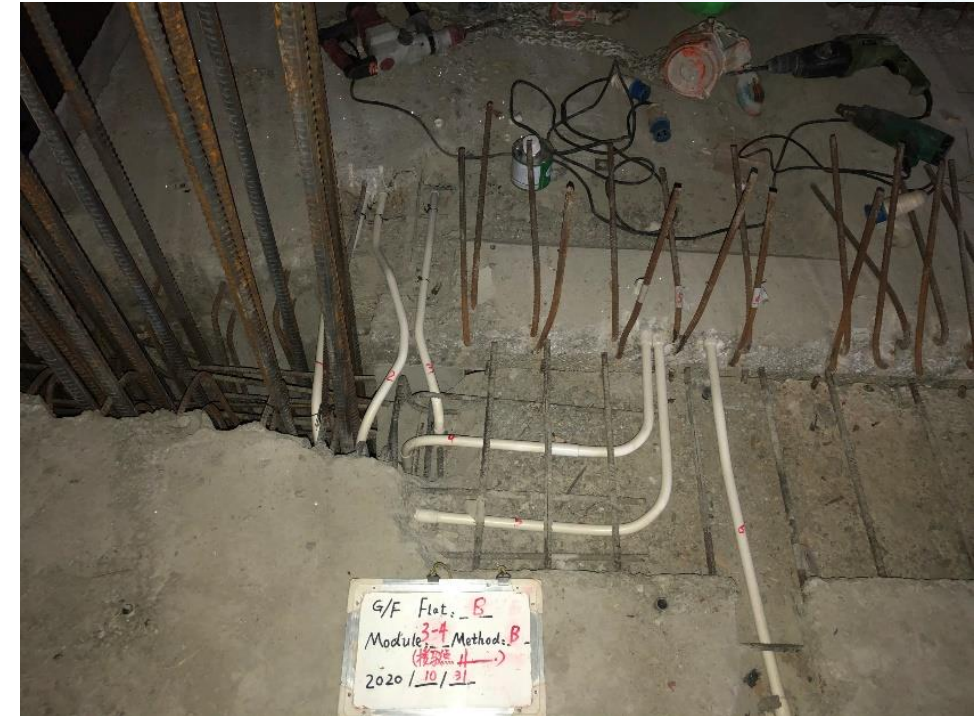
MiC Modules Assembly after conduit connection
