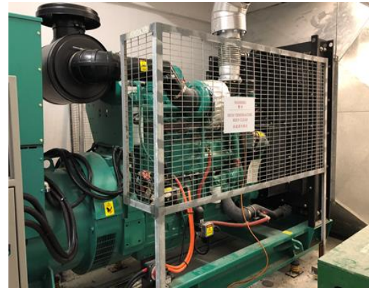
Emergency Generator, Control Cubicle and Switchgear Assembly
