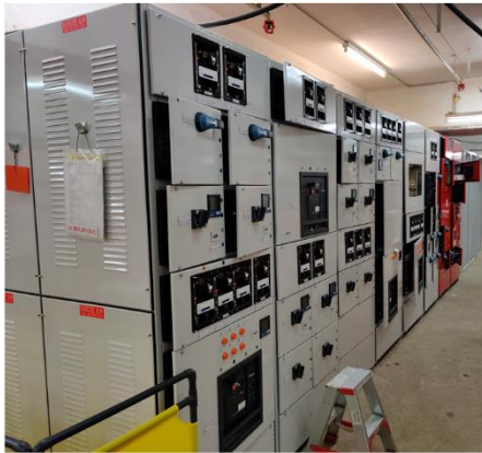
LV Switchboard in Main switchroom
