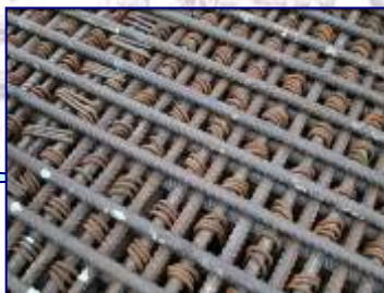
Shear Reinforcement REDUCED
