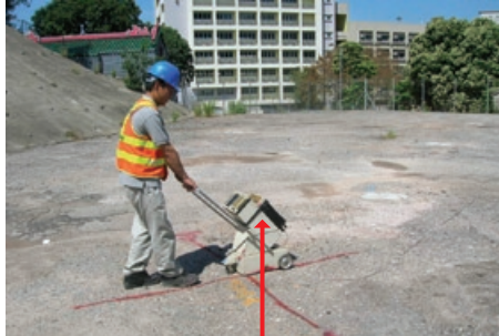
Electronic device to locate underground utilities
