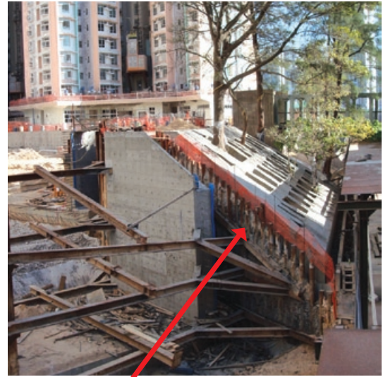
Temporary works for excavation works
