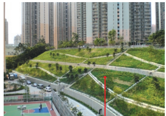
Hydroseeding slope surface protection
