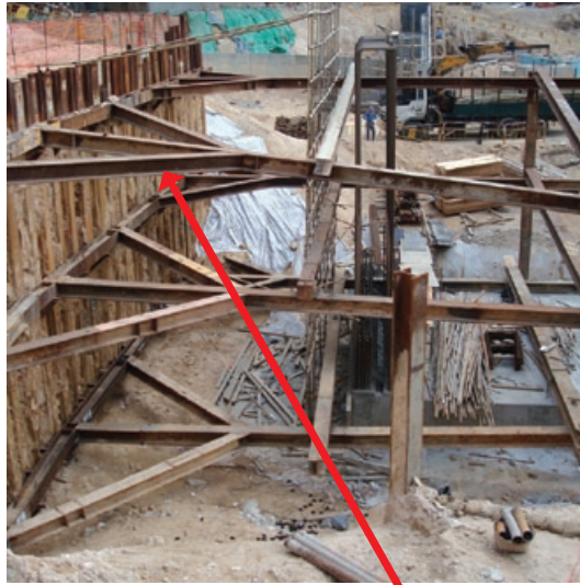
Temporary works for excavation works
