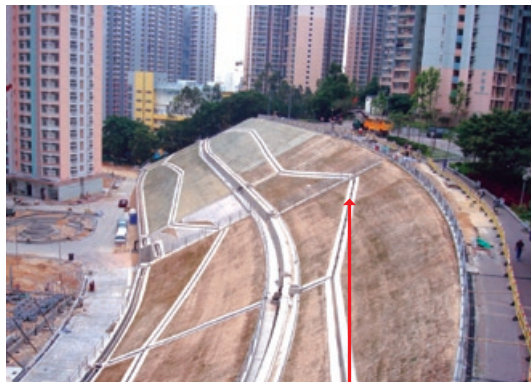
Slope surface drainage system
