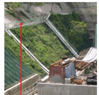
Hand-rail along berm
