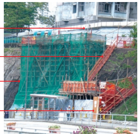
Drilling on a slope
