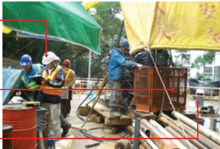
Protection guard & rotary part
