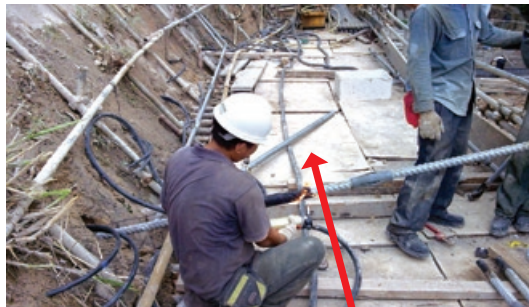
Temporary platform for soil nails works
