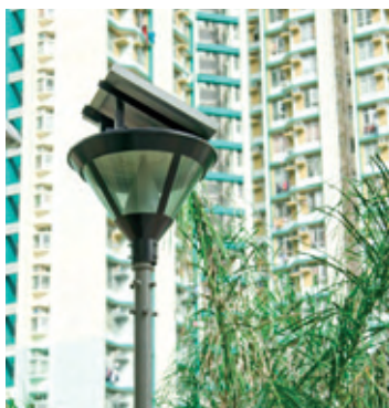
An outdoor lighting system powered by solar energy is under trial at Lam Tin Estate.
