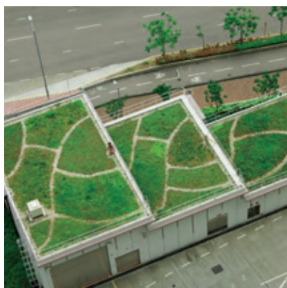
Green rooftops reduce building temperatures while also enhancing the visual appeal.
