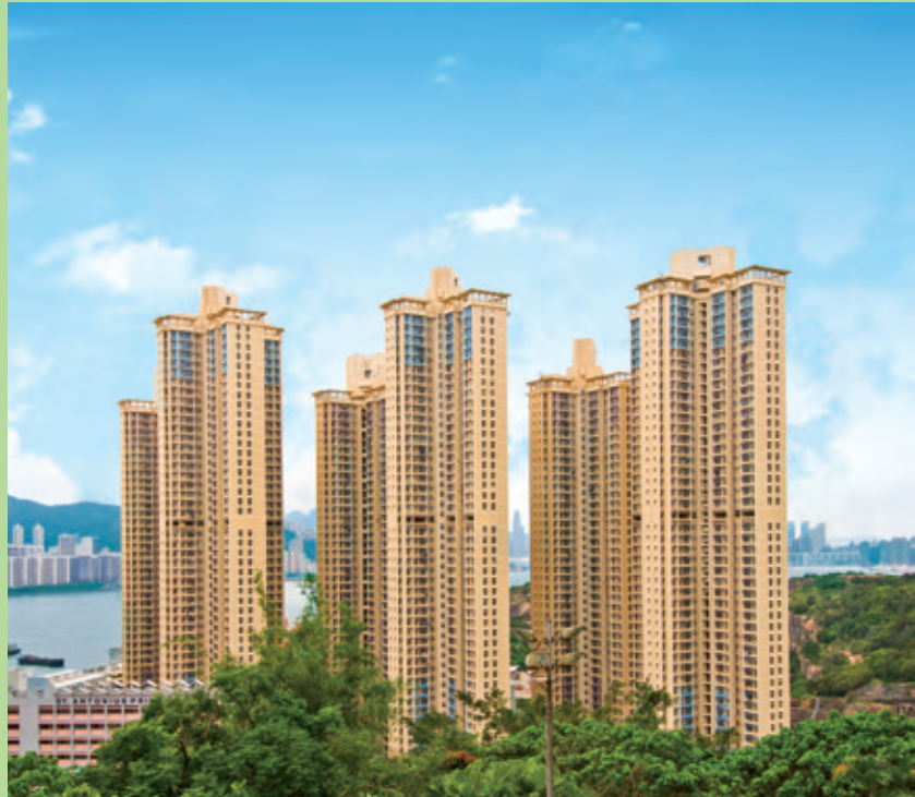
Yau Lai Estate is one of the eight new estates completed this year.
