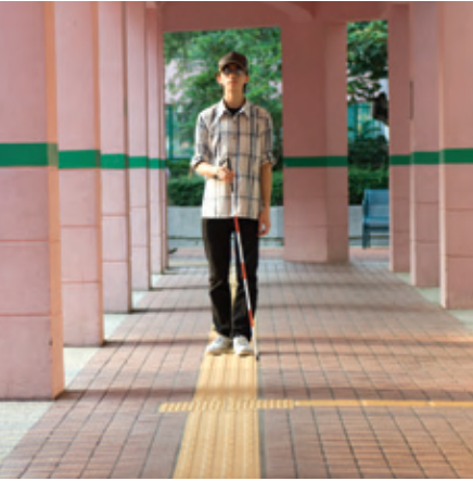
Tactile paths for the visually impaired are part of our Universal Design.
