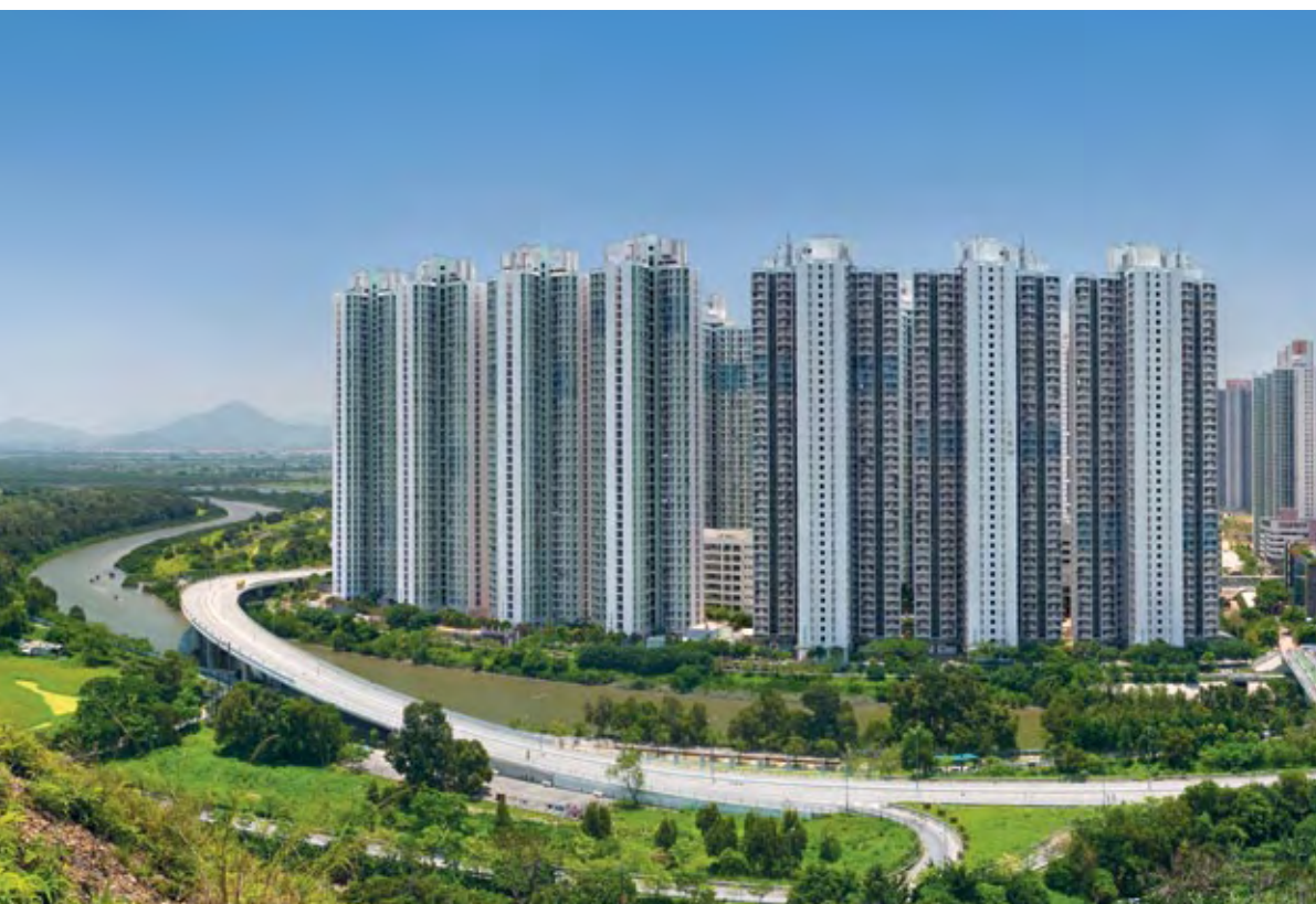
Around 15 000 rental housing units are being built annually to meet the needs for public housing. Picture shows Tin Heng Estate in Tin Shui Wai.
