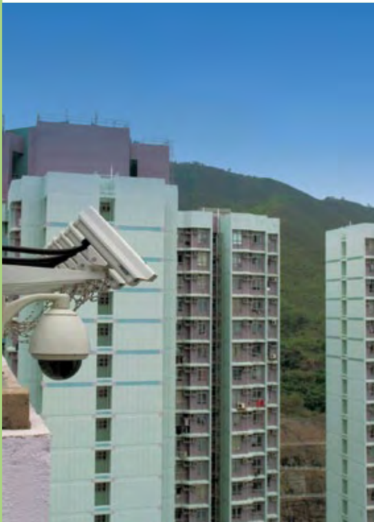
Top: Sai Wan Estate has just gone through the Estate Improvement Programme.
