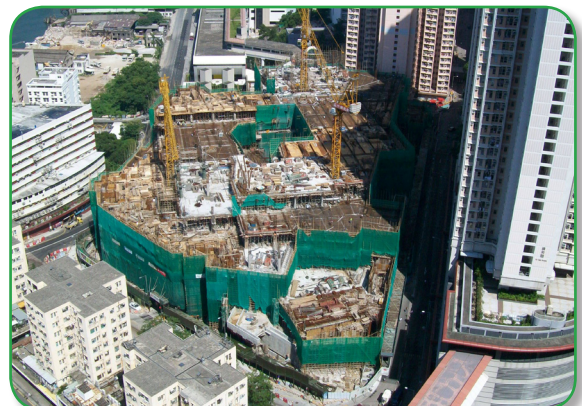
Construction Site of the Domain
