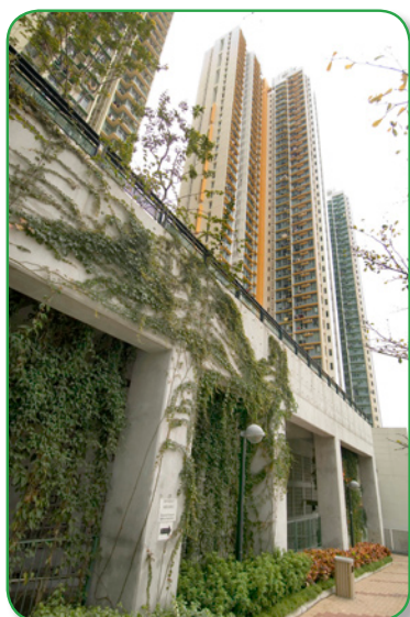
Vertical Green Panels at Yau Lai Estate Phase 4
