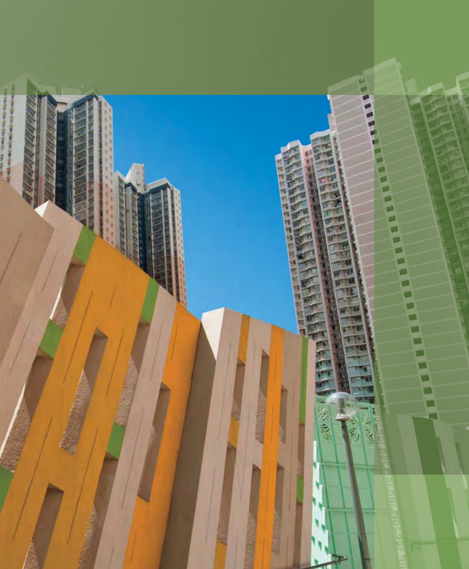
葵涌邨 Kwai Chung Estate
