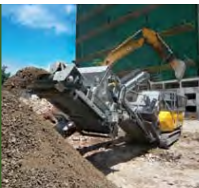
Demolition debris is used for backfilling at building sites.
