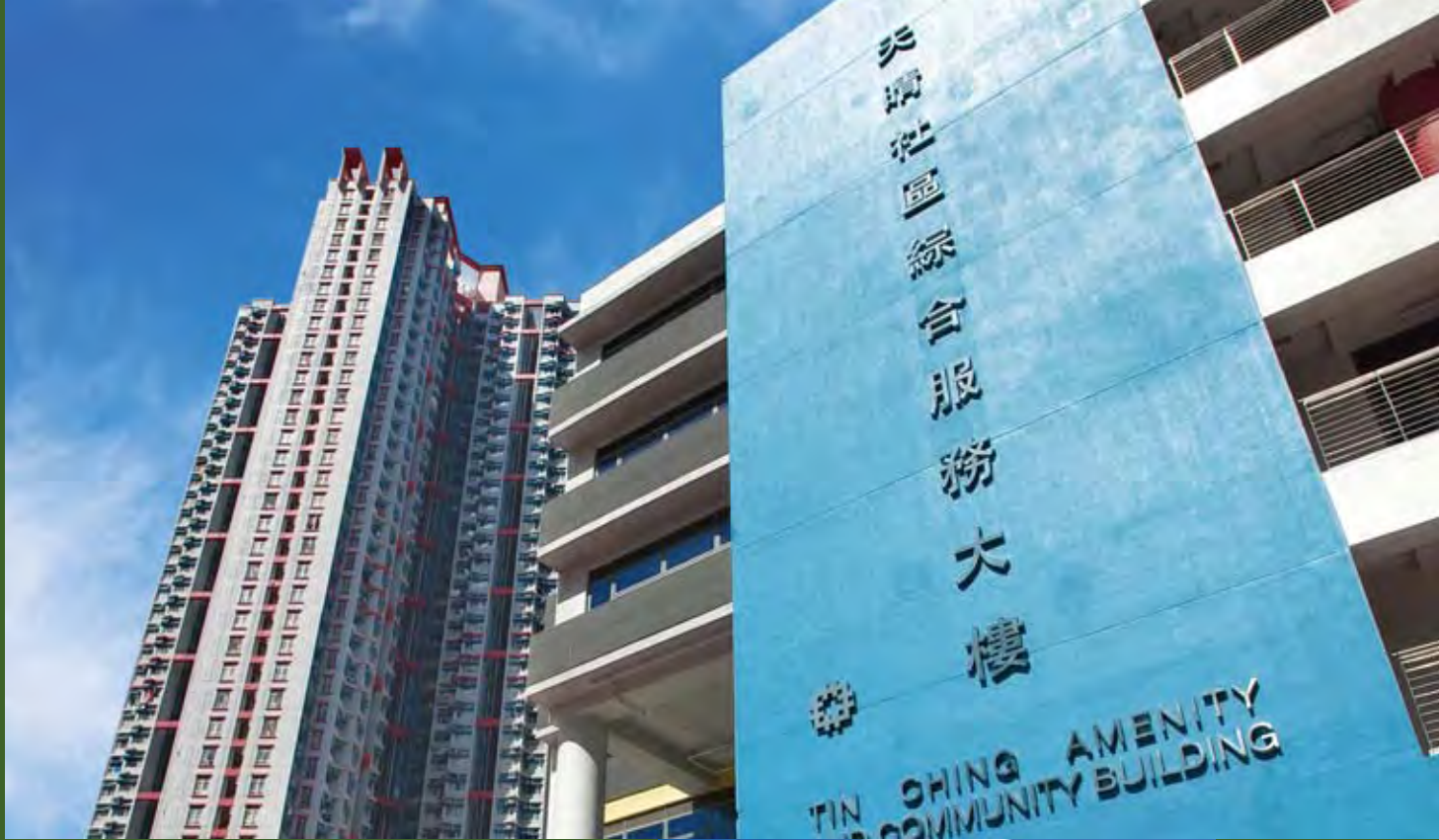
Tin Ching Estate comprises seven residential blocks and the ACB, which has become a social hub for residents of Tin Shui Wai.
