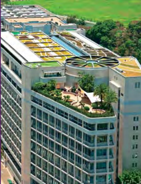
The green roof at our headquarters building demonstrates our green commitment.
