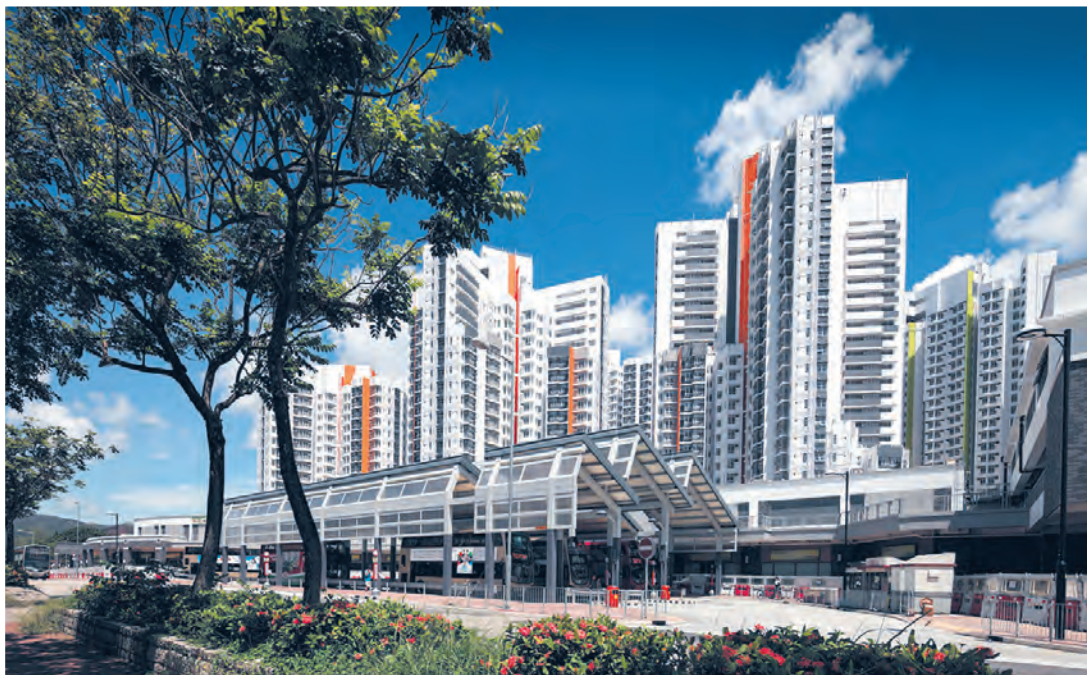
Part of Hung Fuk Estate was completed during the year.
