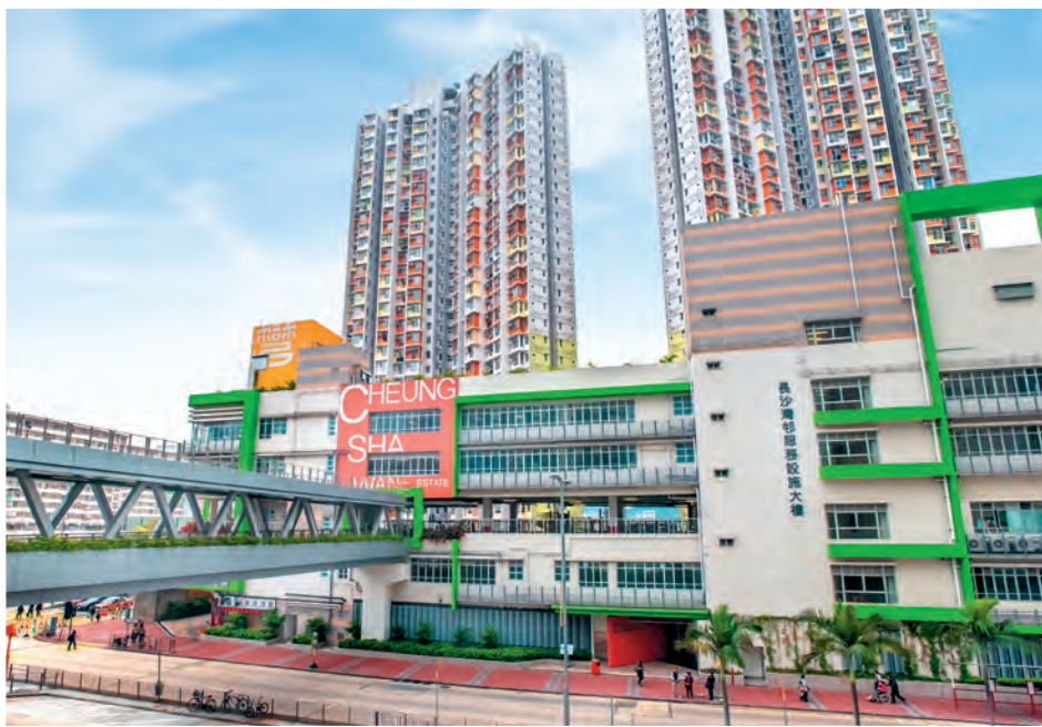
Ancillary Facilities Block, Cheung Sha Wan Estate.
