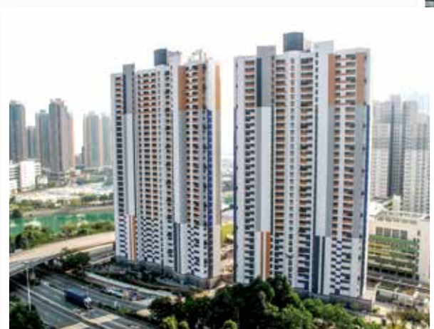
“Single aspect” building design minimises the noise impact of major traffic arteries
