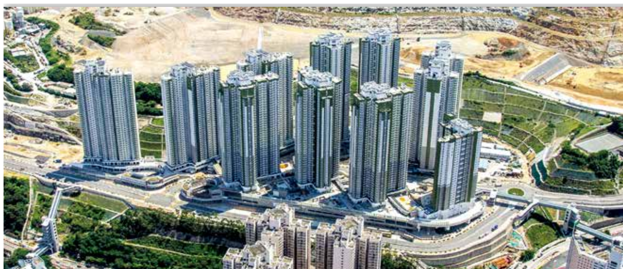
PRH development projects at Anderson Road, Kwun Tong
