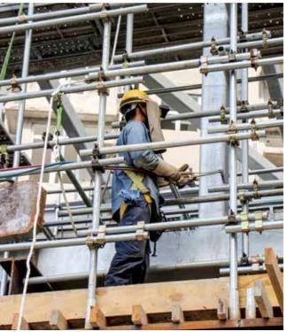
Suitable personal protective equipment is necessary when carrying out welding works
