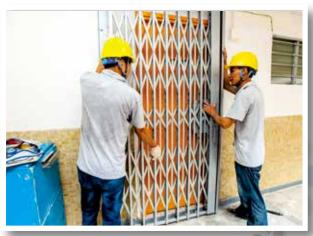
Replacing old type collapsible gates is part of the enhancement programme
