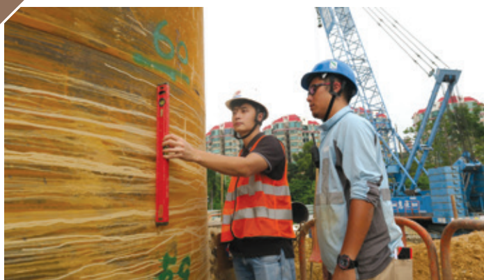
Measuring the verticality of pile steel casing (left) and supervising the construction of driven H-piles to ensure building quality
