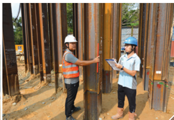
Measuring the verticality of pile steel casing (left) and supervising the construction of driven H-piles to ensure building quality
