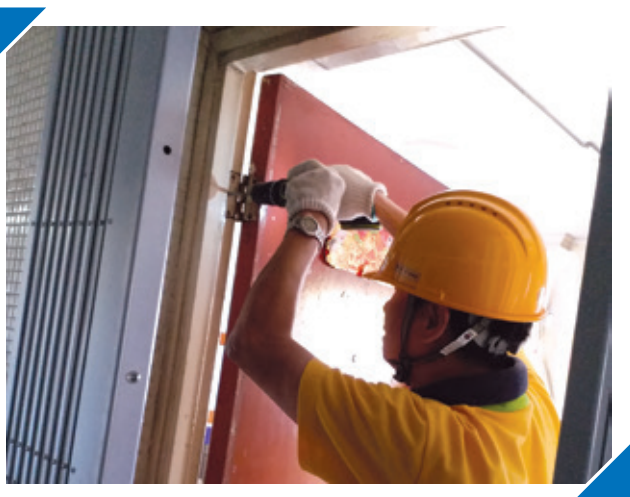
A workman repairs door hinges of a flat under the Responsive In-flat Maintenance Services
