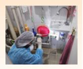
drainage system of all those units that used the same soil pipe and vent pipe. Appropriate repairs to the drain/vent pipe were arranged during the inspection, if necessary.
