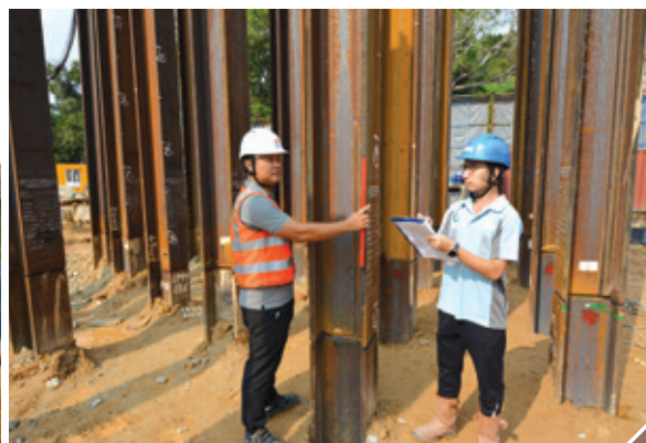
Measuring the verticality of pile steel casing (left) and supervising the construction of driven H-piles to ensure building quality
