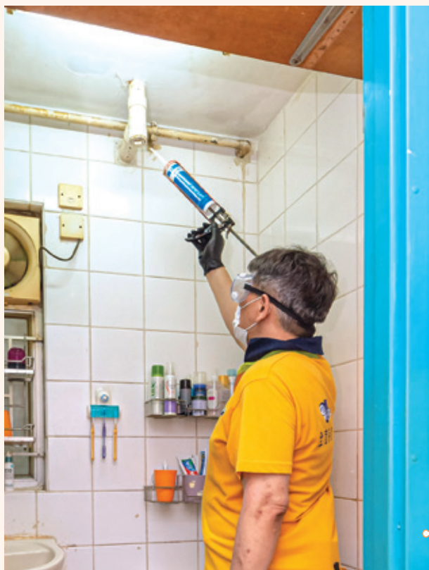
維修慈正邨單位的室內排水管 Carrying out repair work for in-flat drainage at Tsz Ching Estate
