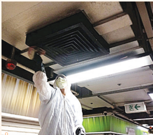
清潔葵涌街市的空調和通風系統 Cleansing of the air-conditioning and ventilation systems in Kwai Chung Market
