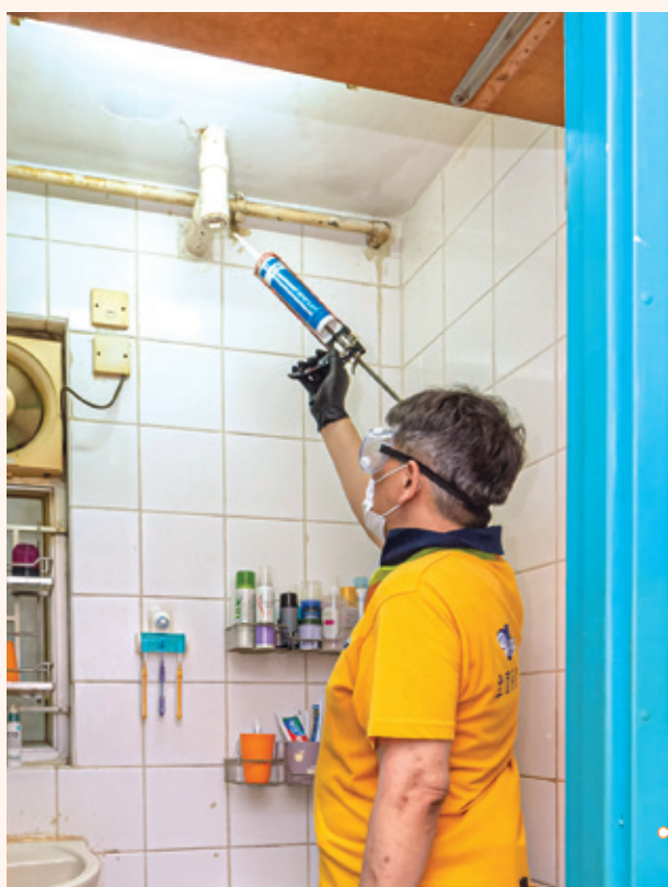
维修慈正邨单位的室内排水管 Carrying out repair work for in-flat drainage at Tsz Ching Estate
