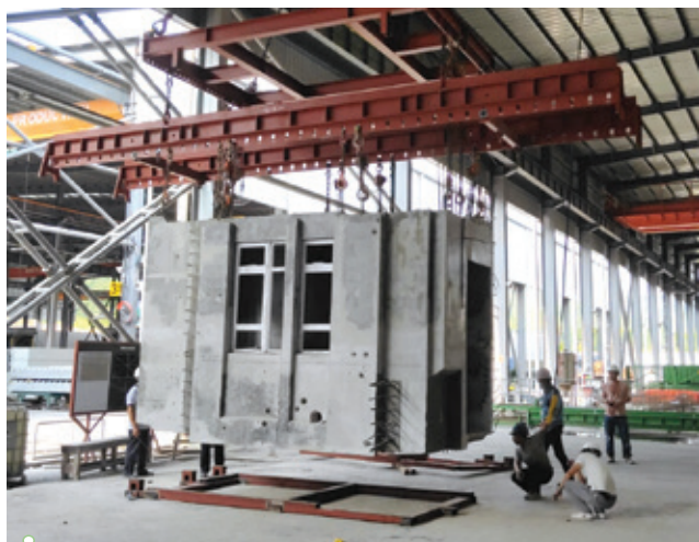
组装合成组件(左)和预制板间墙 MiC modules (left) and precast partition walls
