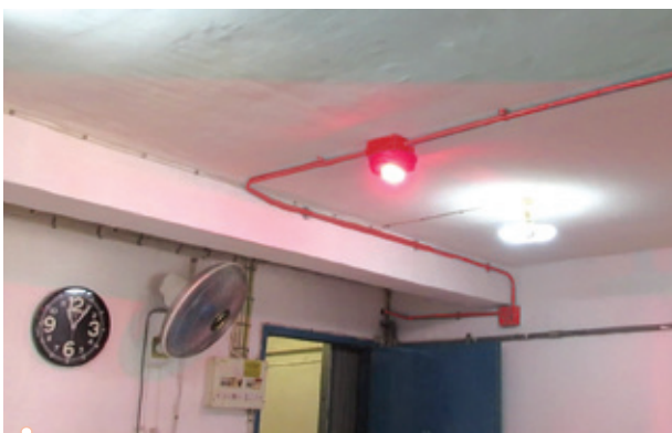
公屋单位内的「火警视像警报系统」闪动 Flashing of a visual fire alarm system inside a PRH flat
