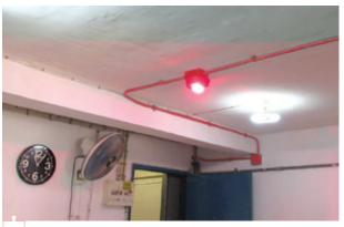
公屋单位内的「火警视像警报系统」闪动 Flashing of a visual fire alarm system inside a PRH flat
