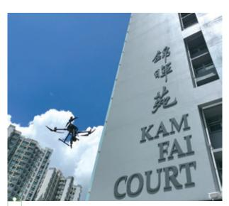
ュニ<sup>ン</sup> 無人機在檢測外牆 UVA inspects external walls of a block
