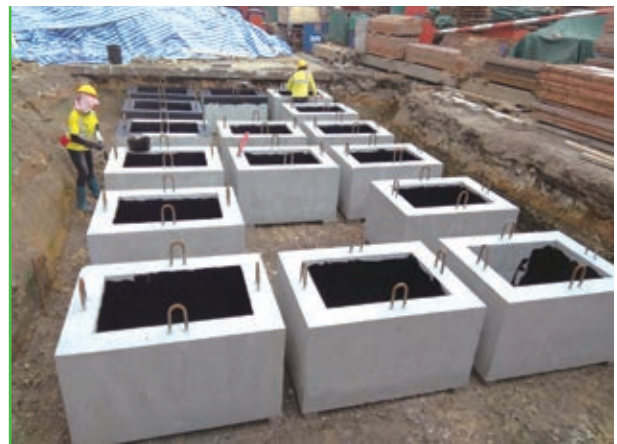
渔湾邨试用构件式零灌溉系统 A trial of modular ZIS at Yue Wan Estate
