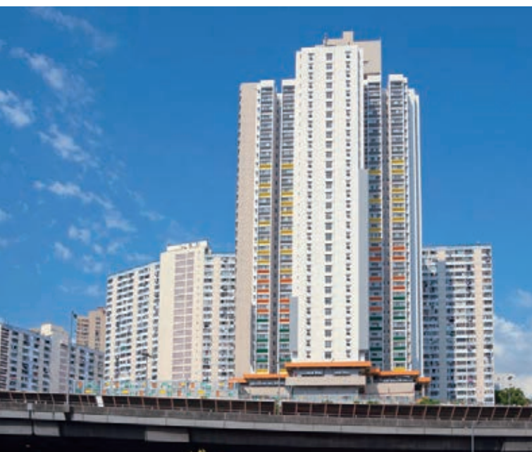
荔景邨恒景樓改裝為社區隔離設施 Heng King House of Lai King Estate is converted into CIF
