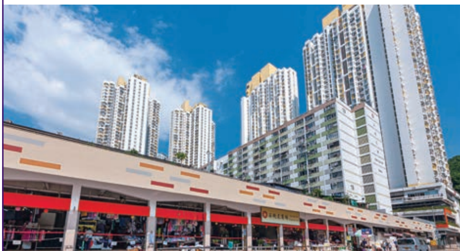
石硖尾街市的外墙改善工程前(上图)后 Refurbishment of external façade of Shek Kip Mei Market – before (top photo) and after
