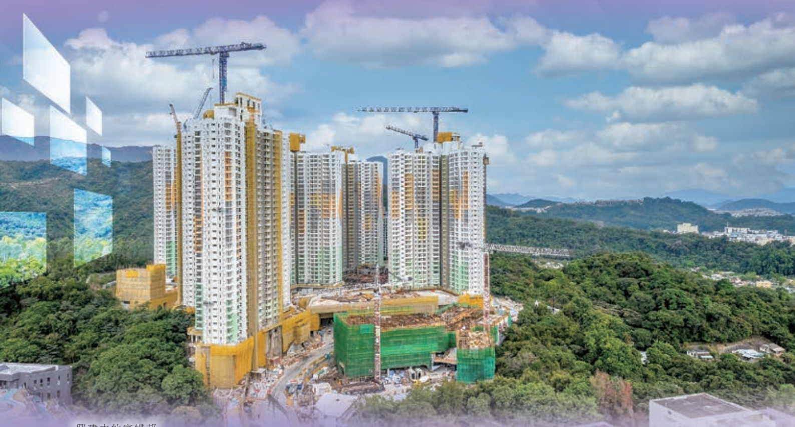
興建中的富蝶邨 Fu Tip Estate under construction
