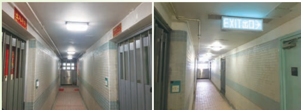
發光二極管凸面照明器 (左圖)和出口指示牌 LED bulkheads (left photo) and an LED exit sign
