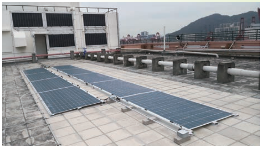
荔景邨的柔性太陽能光伏系統 A flexible PV system at Lai King Estate
