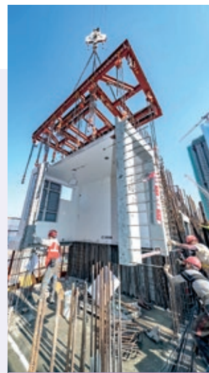
组装合成建筑法大幅减少组装时间 Modular Integrated Construction significantly reduces installation time
