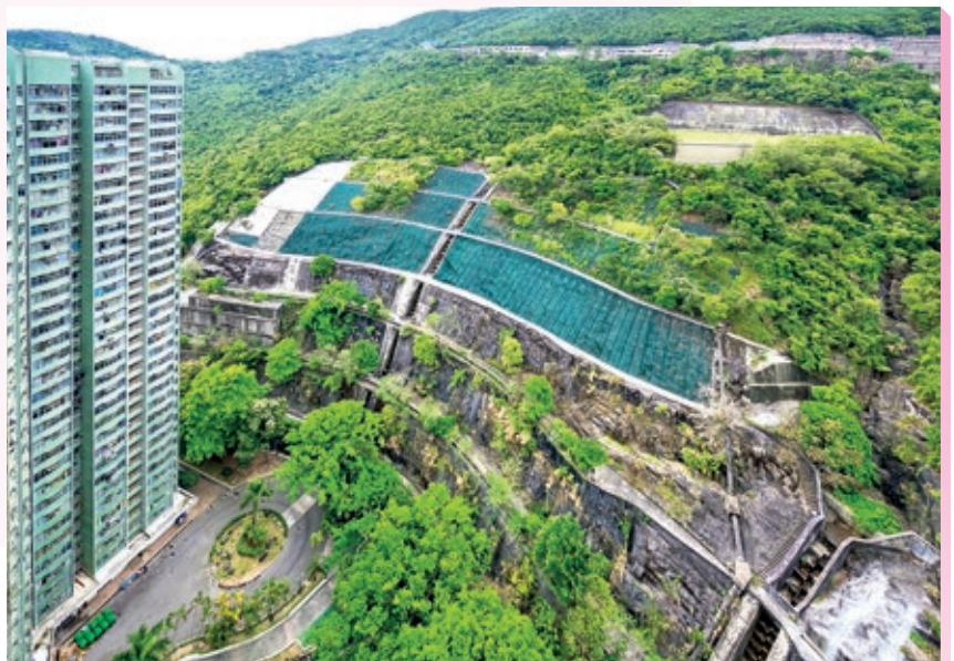
东区小西湾邨斜坡保养工程 Slope maintenance work at Siu Sai Wan Estate in Eastern District
