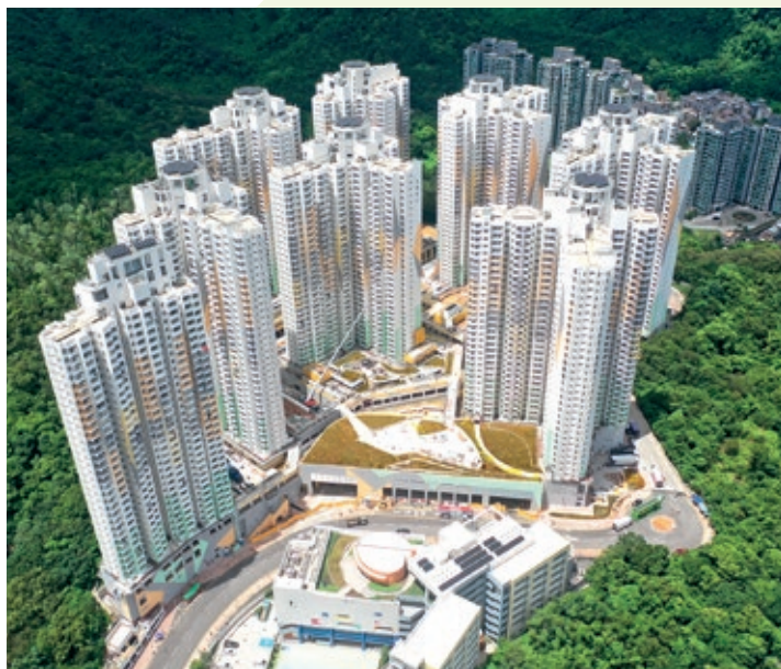
大埔富蝶邨善用布局，在住宅大厦间留下通风走廊，加强自然通风 The domestic blocks at Fu Tip Estate, Tai Po are positioned to form open breezeways for better natural ventilation
