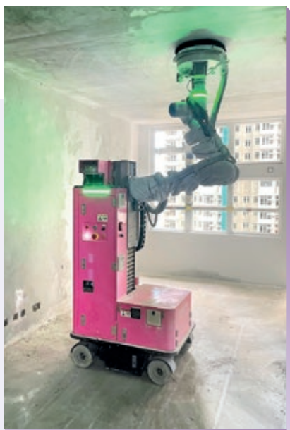
机器人在单位内打磨墙壁和天花 A robot performing wall and ceiling sanding
