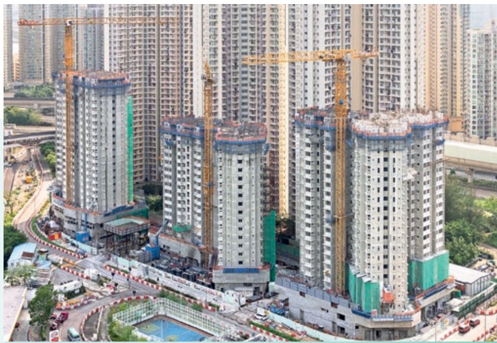
兴建中的马鞍山锦柏苑 Kam Pak Court, Ma On Shan under construction
