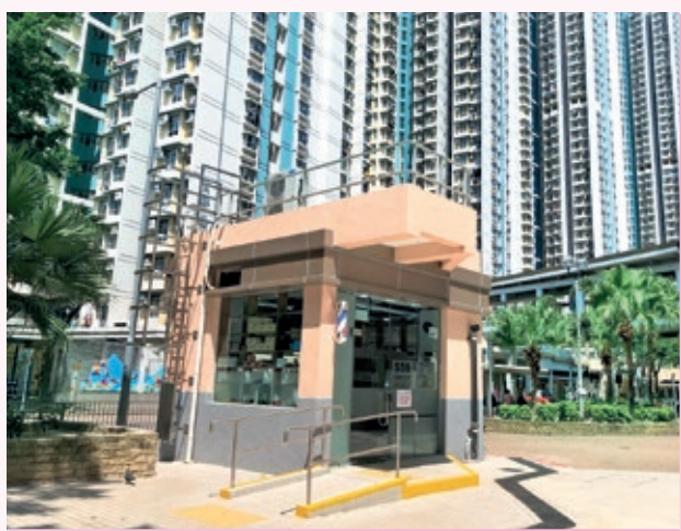
牛头角上邨新增的商铺 A new shop added to Upper Ngau Tau Kok Estate
