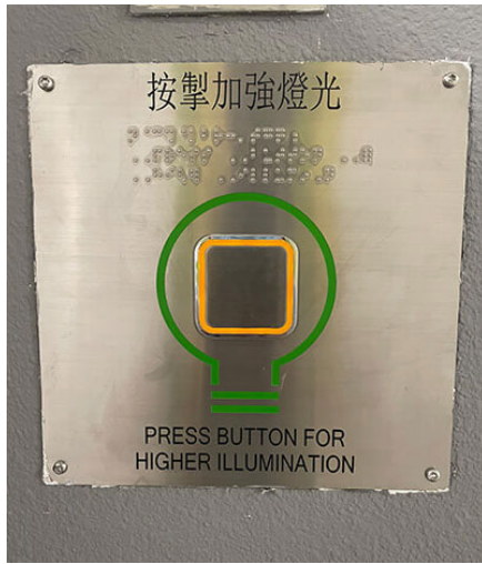
Two-level lighting system
