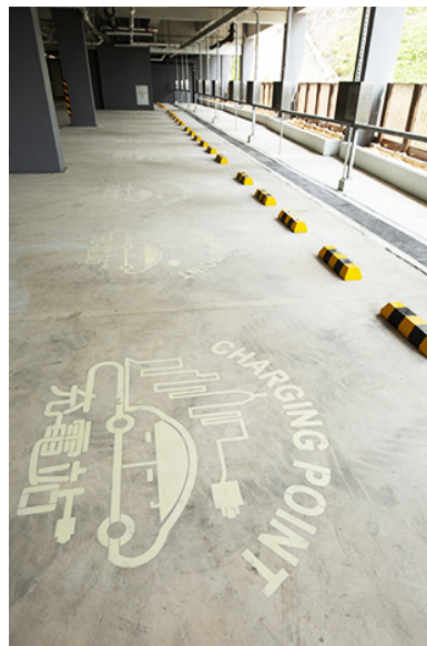
EV charging facilities at Choi Hing Court, Kwun Tong
