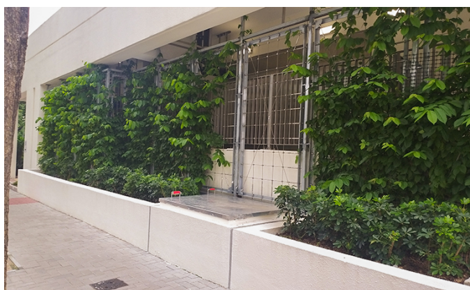
Yue Chun House, Yue Wan Estate
