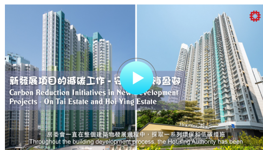
Carbon Reduction Initiatives in New Development Projects - On Tai Estate and Hoi Ying Estate
