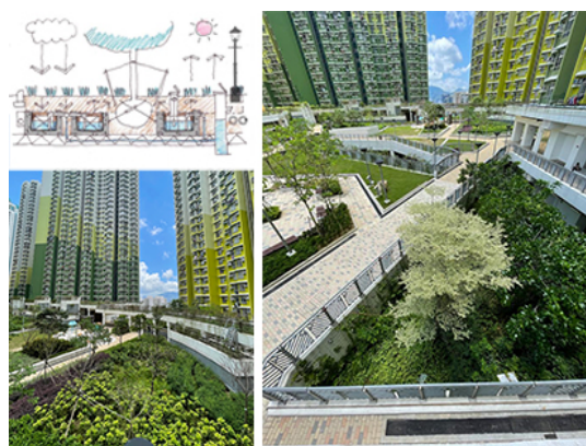
Zero Irrigation System in the stepped planters are adopted to reduce the consumption of potable water.
