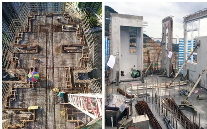
Precast elements during building construction
