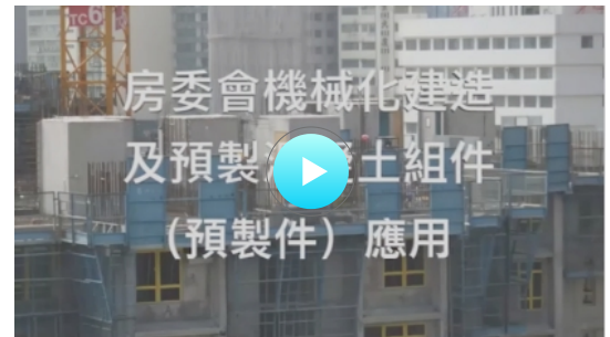
Precast concrete construction
