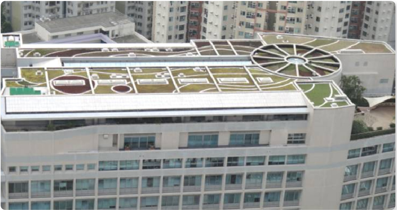
Green Roof at Housing Authority Headquarters
