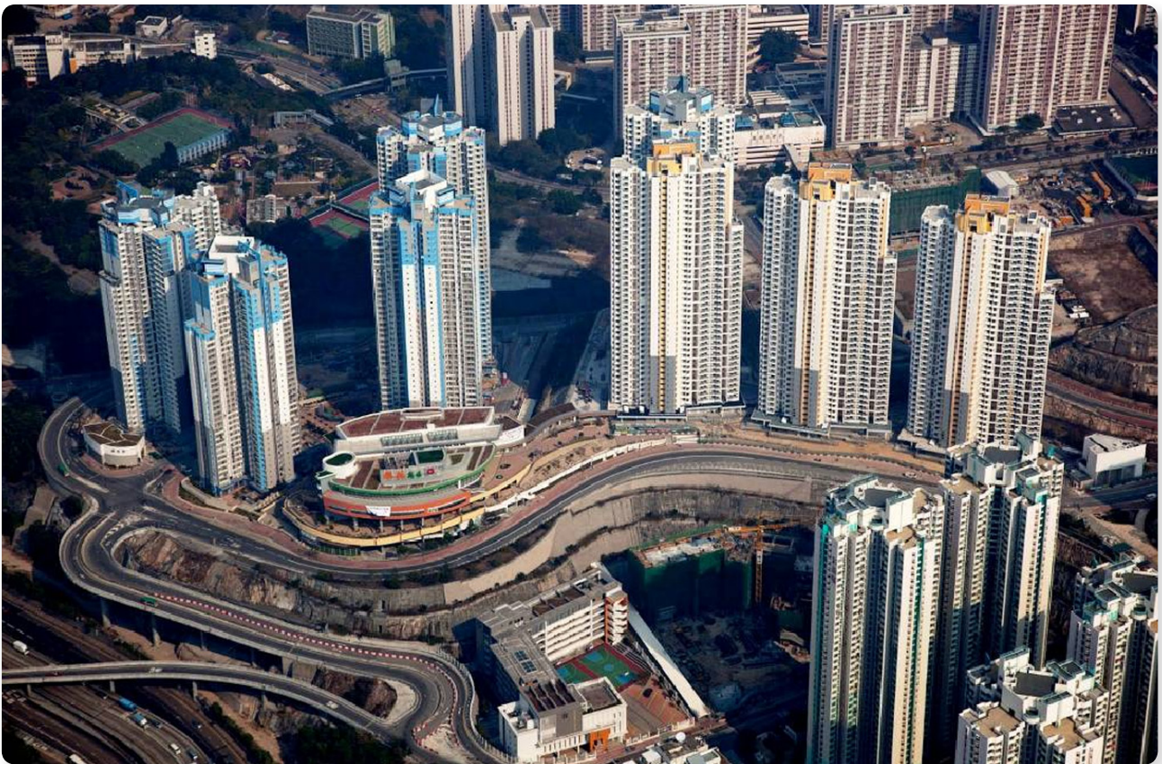
Choi Tak Estate – Newly Completed Estate Using Micro-climate Study
