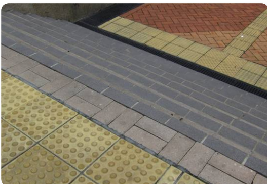
Tactile Warning Strips on Landings at the Top and Bottom of Staircases
