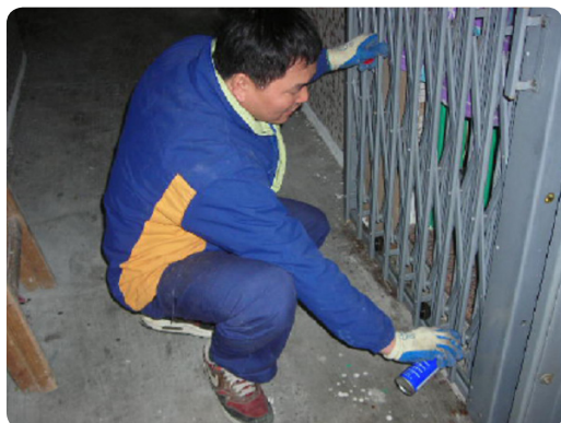
TMS – On-site Maintenance
