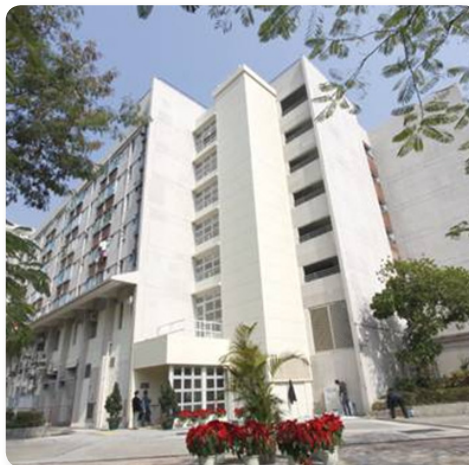
Lift Installation in Shui Pin Wai Estate
