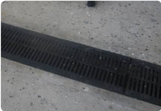
Gratings or Cover in Surface Channel
