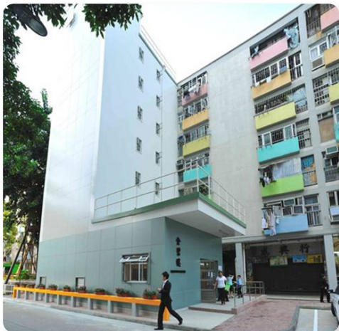
Lift Installation in Choi Hung Estate
