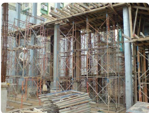
Metal Scaffolding for Double Deck Walkway
