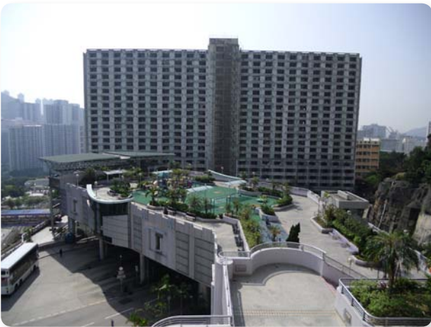
Interim Housing at Block 12 Kwai Shing East Estate
