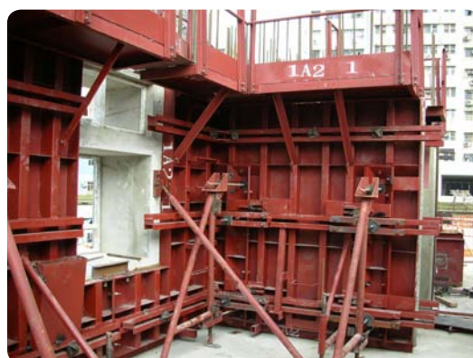
Large Panel Formwork
