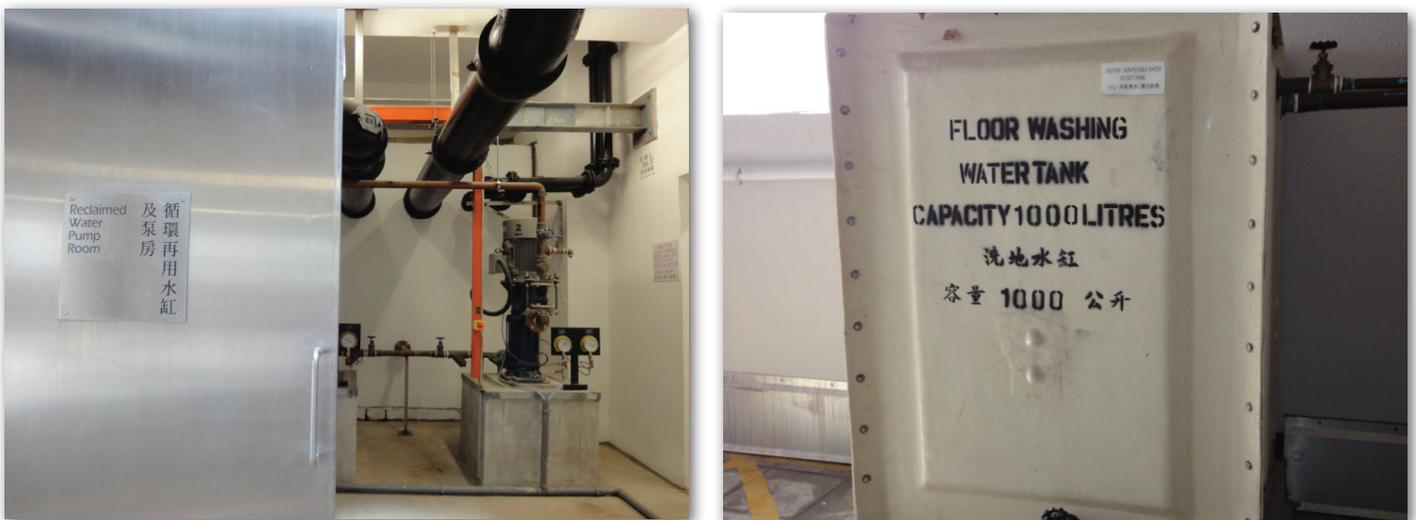
Rain Water and Air Conditioning Condensate Water Harvesting System
