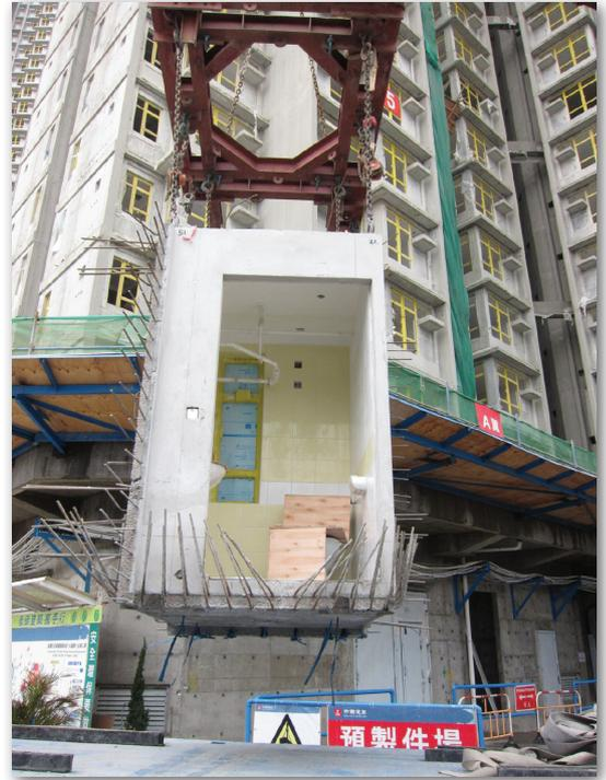
Volumetric precast bathroom
