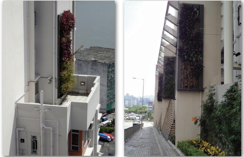
Vertical green panels installed at roof and noise barrier
