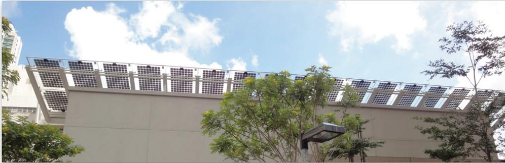
Building Integrated Photovoltaic Panels
