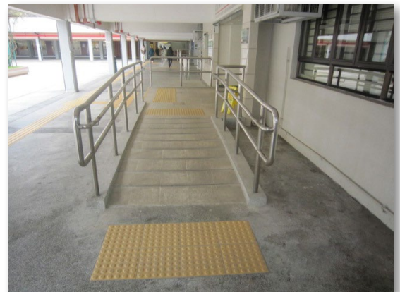
Ramp for persons with disability
