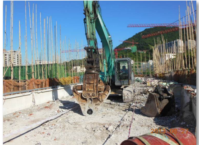
Employing hydraulic concrete crusher at site
