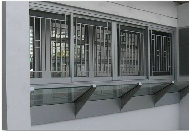
Acoustic balconies and architectural fins
