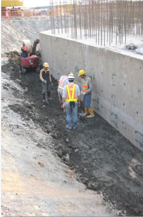
Use of cement-stabilised marine mud for backfilling
