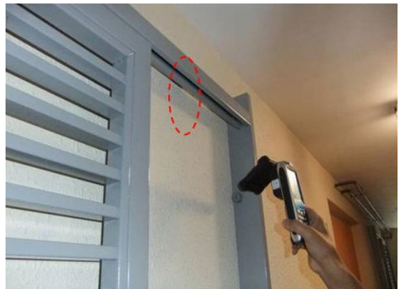
Use of RFID for metal gateset identification
