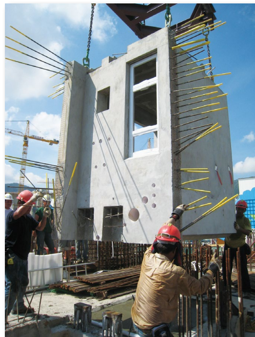
启德第一乙区的立体预制浴室
